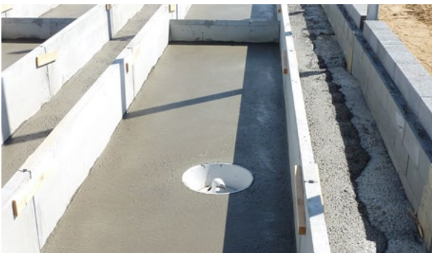
Seamless stud casting of sump module and therefore time-saving. The sump module is adjustable, providing quick change of sluice rate
