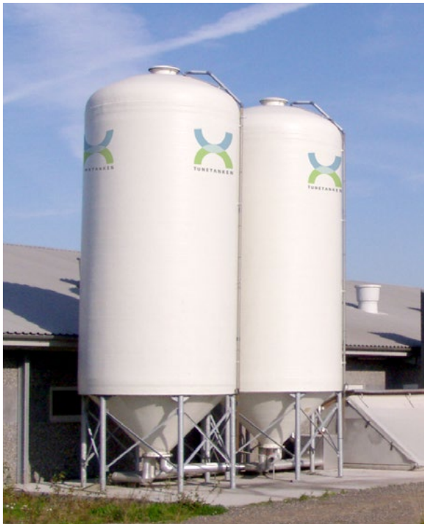
Tunetanken whey tanks with 45° cone bottom.
